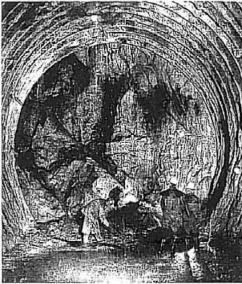
Figure 21: Use of lattice girders with shotcrete in the Monastero pressure tunnel, Italy 1958 (Curzio 1963)
