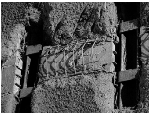
Figure 9: Detail of an HDC element installed between the TH ribs.
