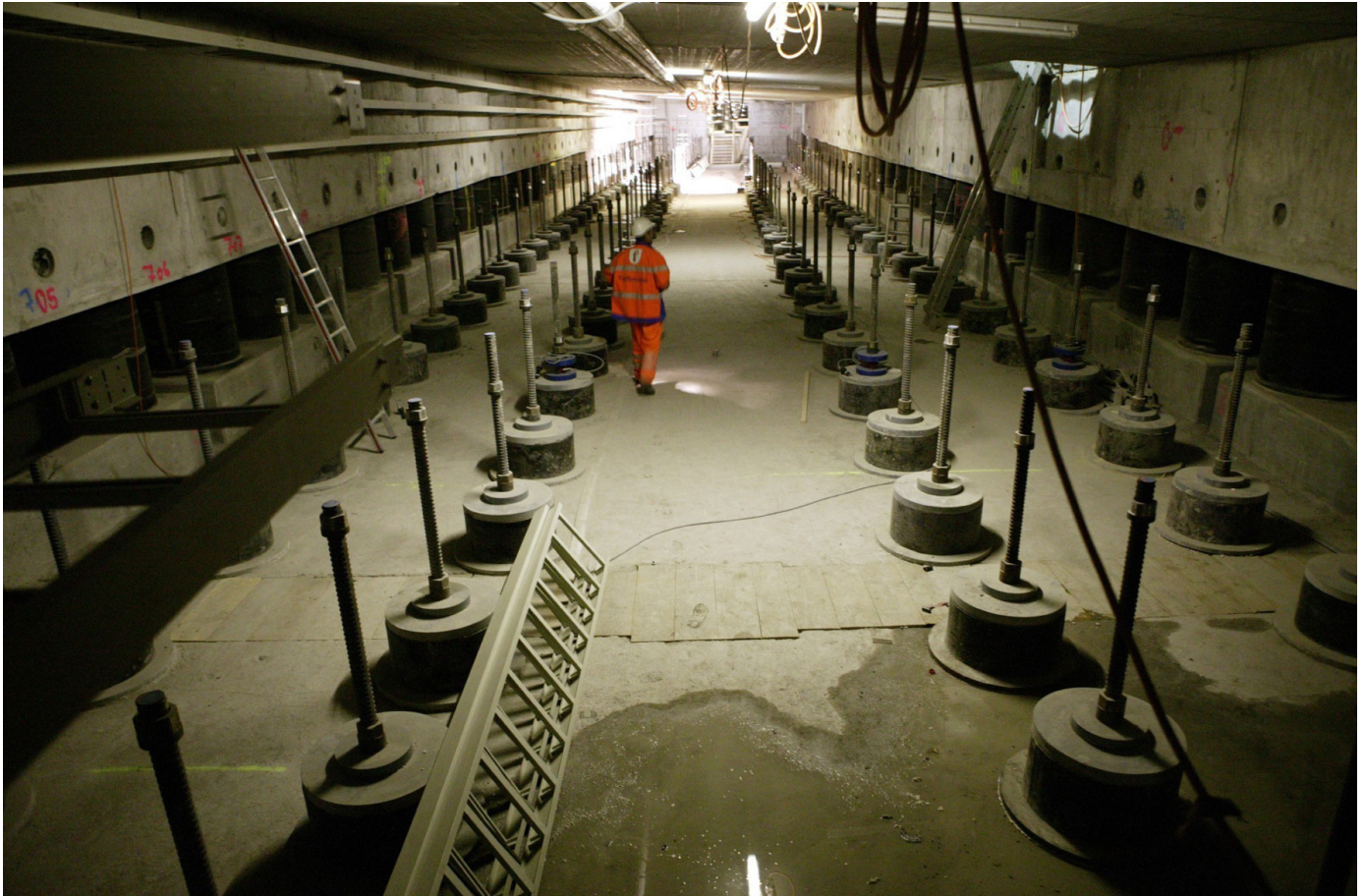
Figure 6. The free space under the carriageway
